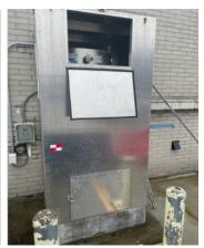
FSEs are required to use the PDX Cooking Oil Removal System, which requires the proper tools and equipment when handling large amounts of fryer oil. This minimizes spills and hazards when transporting liquids to external storage areas. FSEs with fryers are equipped with a fryer oil recovery system which transports fryer oil directly from the FSE to the large storage tanks. Tanks are pumped out on an as needed basis. Recycled fryer oil returns to PDX as biodiesel which fuels aircraft.
