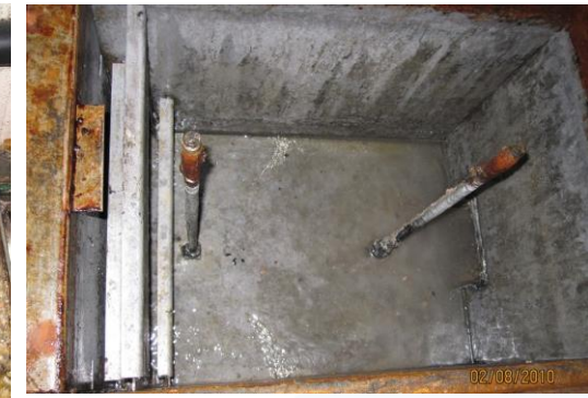
Interceptor pumped out - cleaned to standards.
