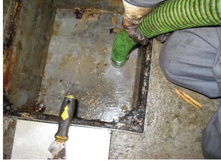
Oversee contractors for complete, correct service.
