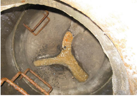
Grease from first dishwasher cycle.
