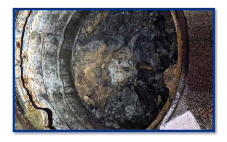
A neglected grease trap resulted in extreme mold overgrowth and foul odors.
